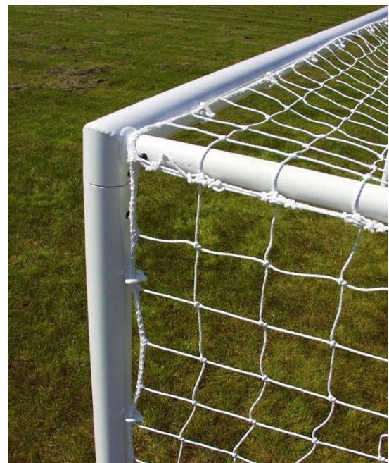
This shows you the hooks on the goals. You simply attach the net over the hook. These are attached on both field 4 & 5
